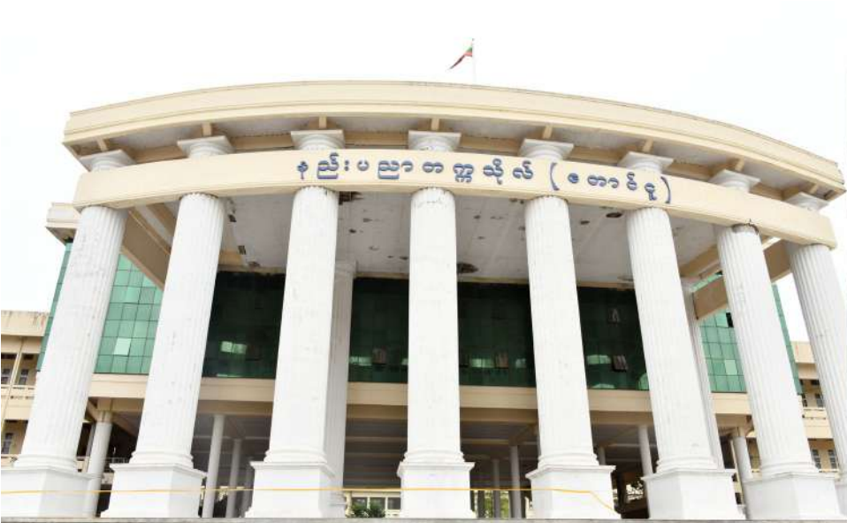
Vice-Senior General Soe Win visits Taungoo Technological University to inspect damage caused by the earthquake.
