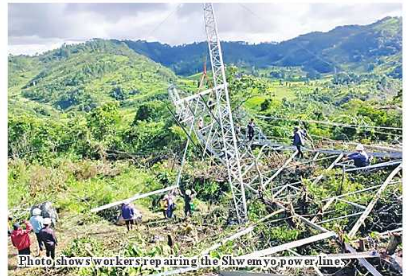
Workers repairing the destroyed pylon 105.
