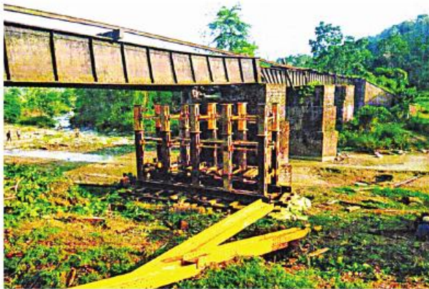
Photo shows the 120-foot long bridge No. 555 on the Myitkyina-Mandalay railroad blown up by KIA.
