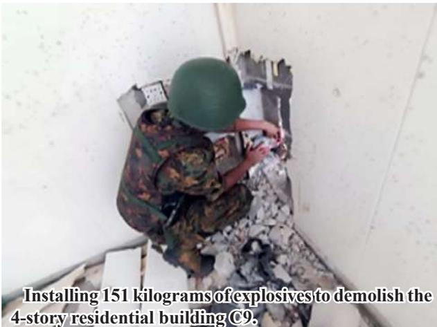
Installing 151 kilograms of explosives to demolish the 4-story residential building C9.
