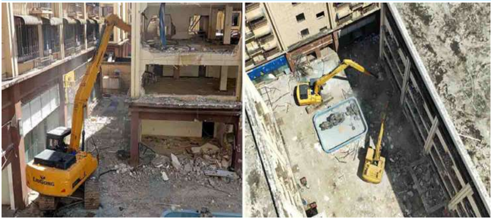
Demolition underway using heavy machinery.
