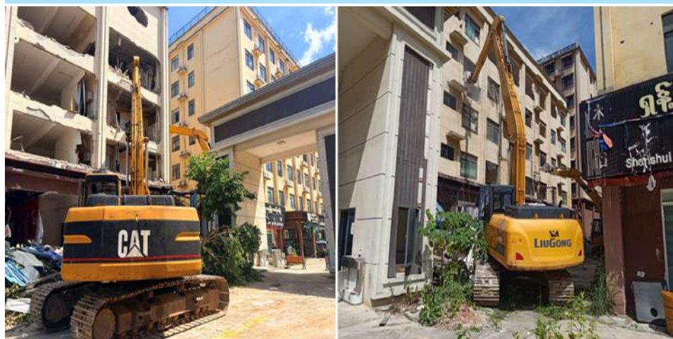
Demolition using heavy machinery.
