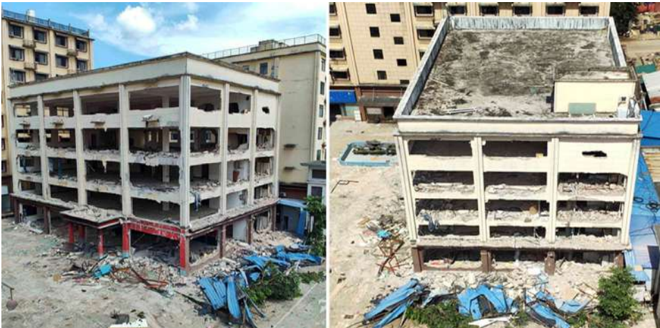
Completion of the demolition.
