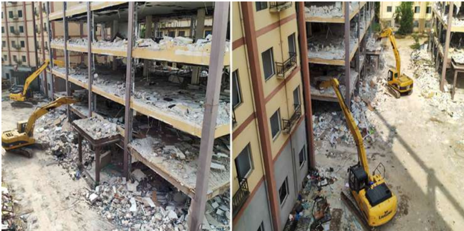
Demolition using heavy machinery.
