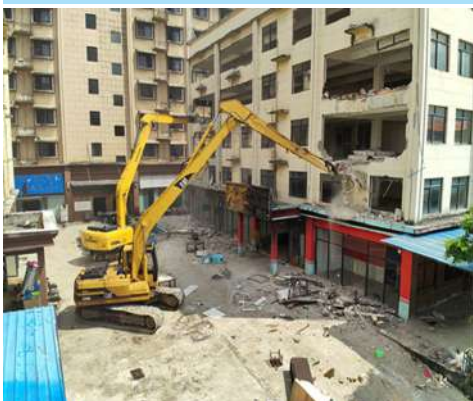
Demolition using heavy machinery.
