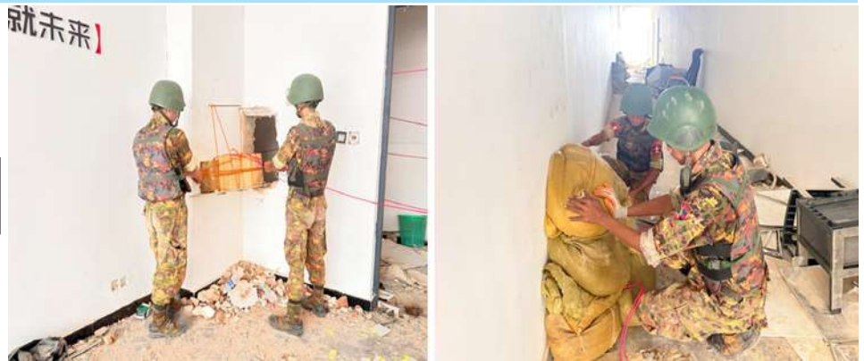
The process of preparing and rigging explosives.
