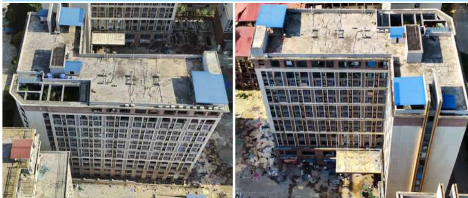
The 13-story building being rigged with explosives.
