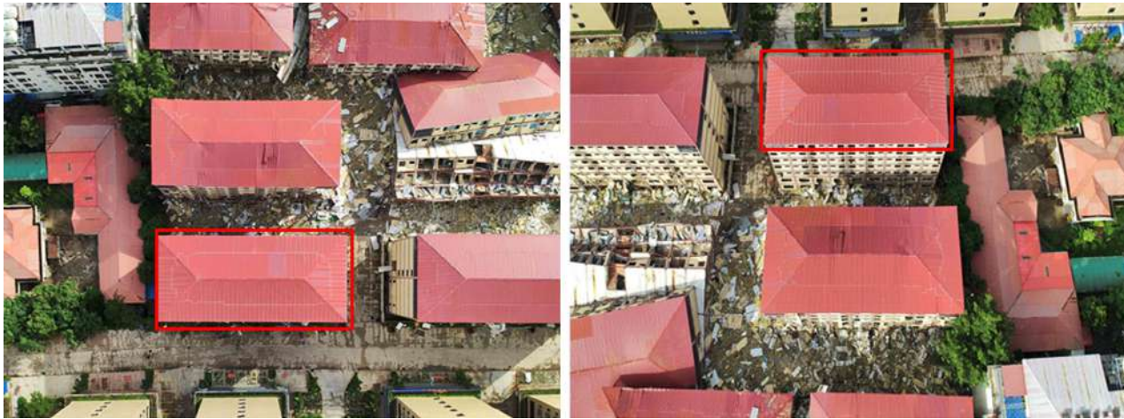
Before the demolition of an illegal 7-story residential building used for online gambling fraud operations in the Shwe Kokko area, Myawaddy District, Kayin State.
