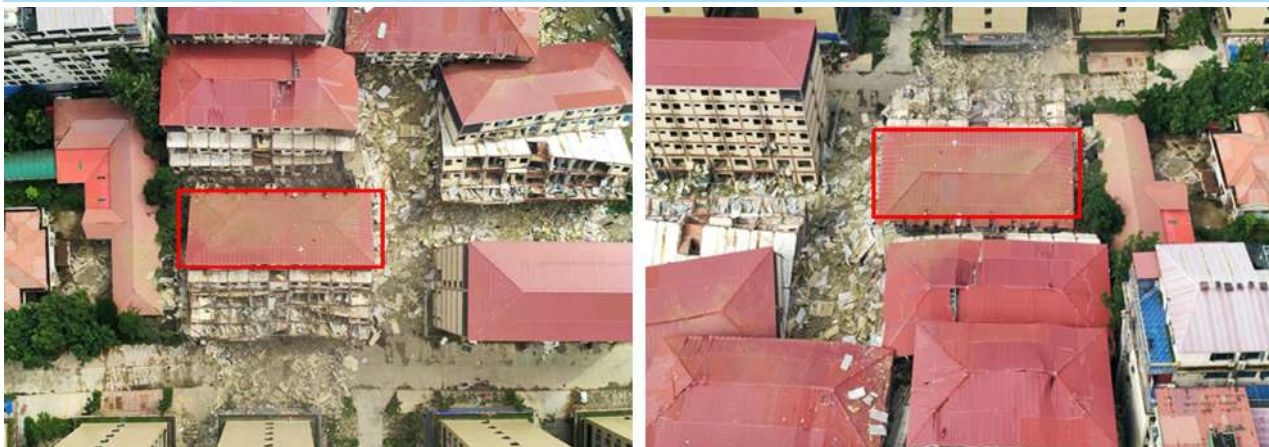
After the controlled explosion and demolition of the illegal 7-story residential building used for online gambling fraud operations in the Shwe Kokko area, Myawaddy District, Kayin State.
