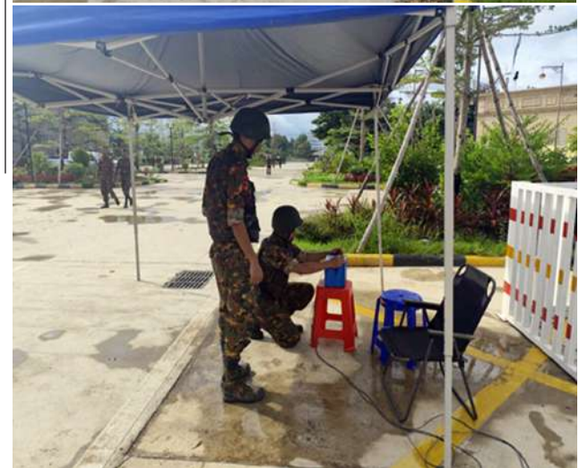
Preparations underway to demolish an illegal 7-story residential building with explosives, which was used for online gambling fraud operations in the Shwe Kokko area, Myawaddy District, Kayin State.
