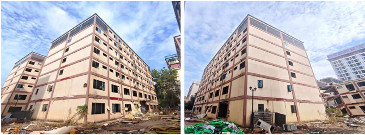
Before the demolition of an illegal 7-storey residential building in Shwe Kokko, Myawaddy District, Kayin State, which had been used for online scam gambling operations.
