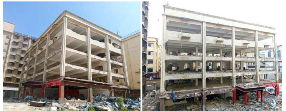
Completion of demolition.
