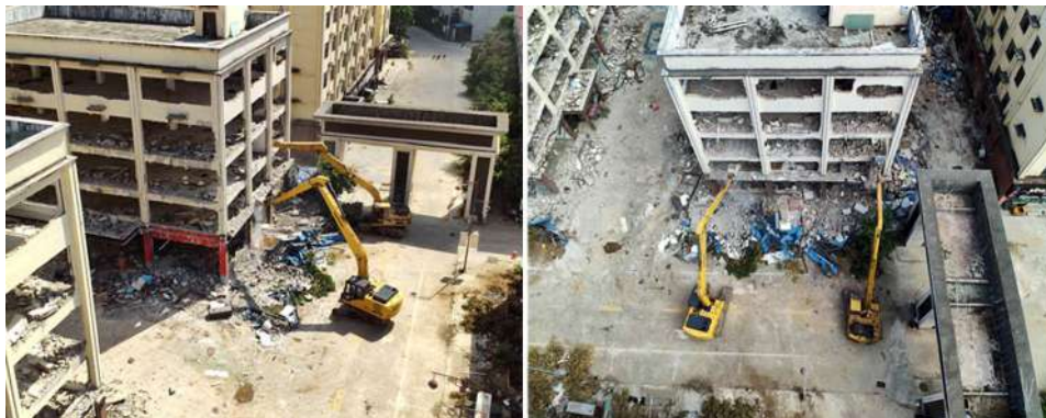
Demolition using heavy machinery.
