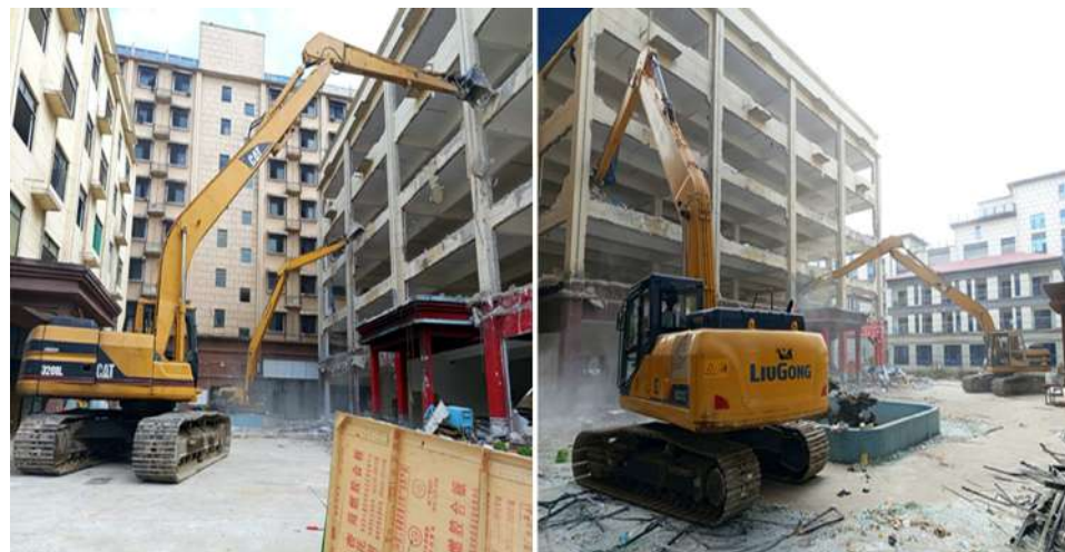
Demolition using machinery.
