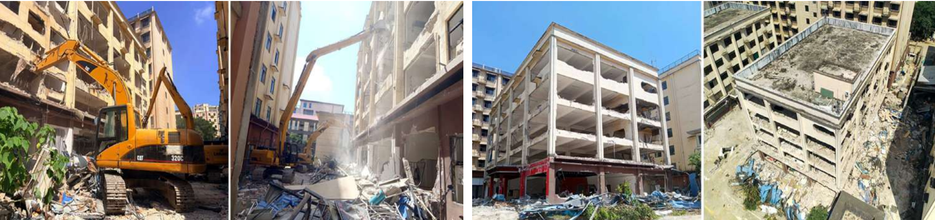
Demolition using heavy machinery.
