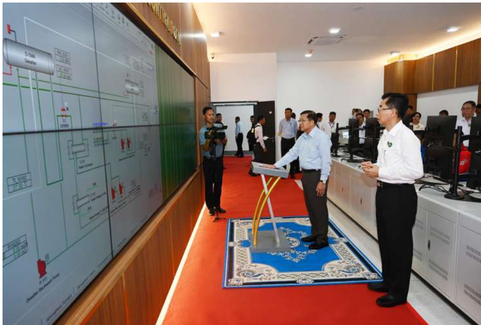
President U Min Aung Hlaing pushes the digitalized button to send raw material and start the engines in the main control room.
