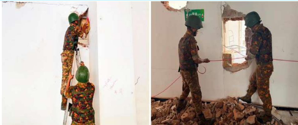
The process of preparing and rigging explosives.
