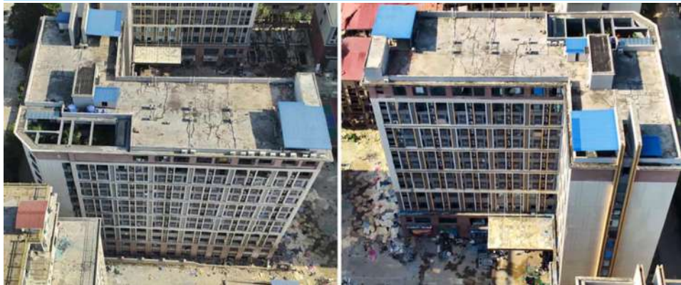
The 13-story building being rigged with explosives.
