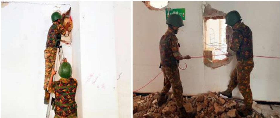
Rigging and attaching explosive charges.
