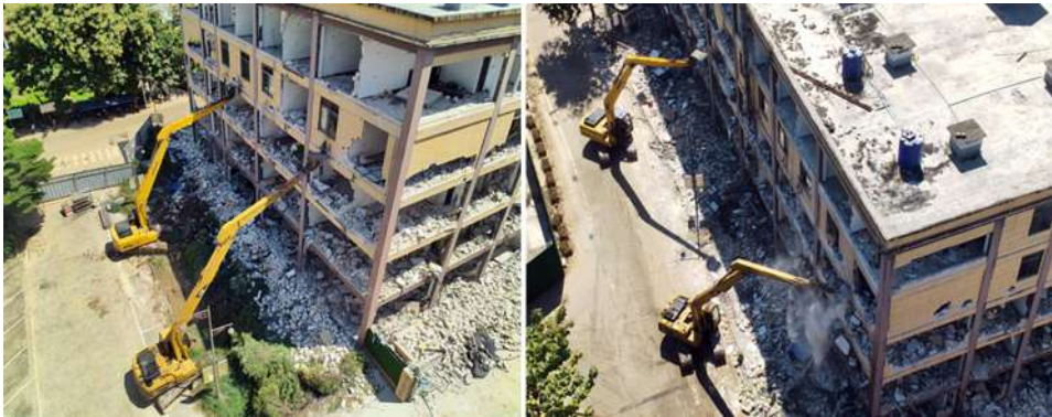
Demolition using heavy machinery.
