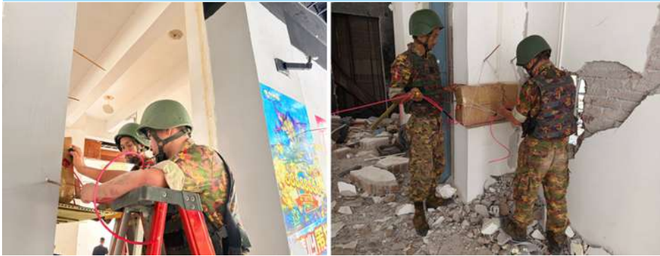
Setting up and planting explosive charges.
