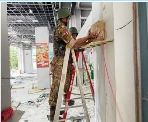
Preparing and setting explosive charges.
