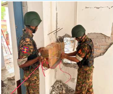
Preparing and setting explosive charges.
