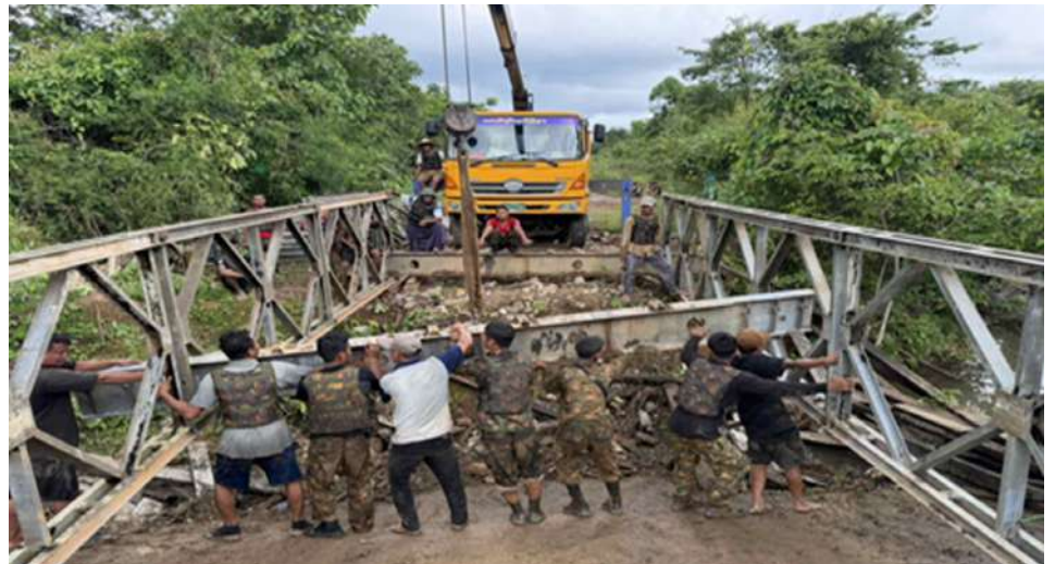
Record of reconstruction of the 30-foot steel-truss Bailey bridge at Mile-40 Bridge, destroyed by terrorist insurgents.
